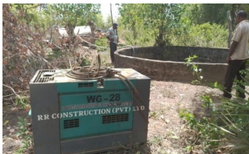
Figure 1- Water pumping from wells to bowser; these facilities provided by Contractor
