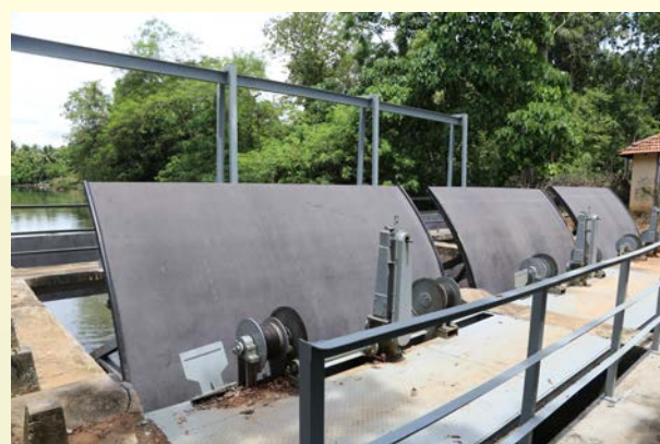
Hydro Mechanical Works of Walawa RB Canal
