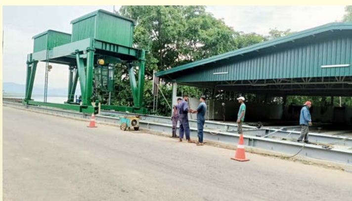
Gantry Crane at Udawalawe Dam
